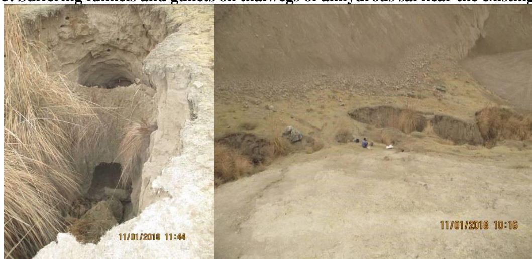
Fig. 5. Suffusing funnels and gulleets on thalwegs of anhydrous sai near the existing road
