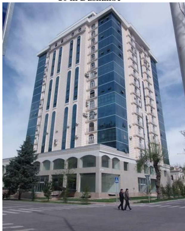
Fig. 1. General view of the erected high-rise residential building on the street. Pushkin, 10 in Dushanbe
