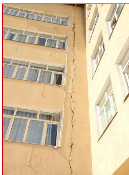
Figure 1. Deformation of the building (a) and roads (б, в) on the campus
