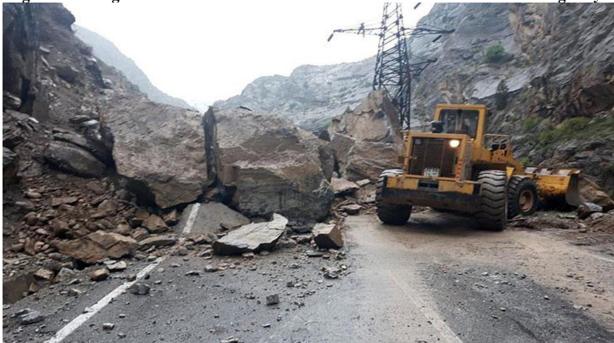
Figure 2. Falling of rubble in the 94-95 km section of the Vahdat-Rasht-Lakhsh highway
